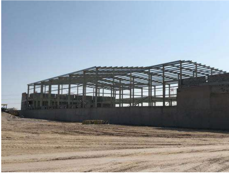
Construction of Warehouses, Accommodation, Offices, Showrooms for Noble Warehousing Co.
