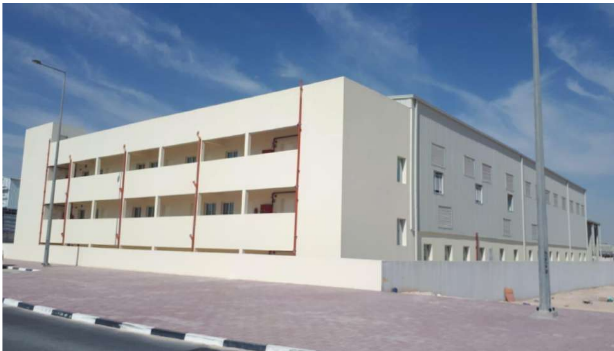
NOBLE WAREHOUSING COMPANY (SHOWROOM, OFFICE, STORES AND ACCOMMODATION) AT BIRKAT AL AWAMER. OWNER: YOUSSEF AL MUSLAH TOTAL PROJECT COST 6,630,000.
