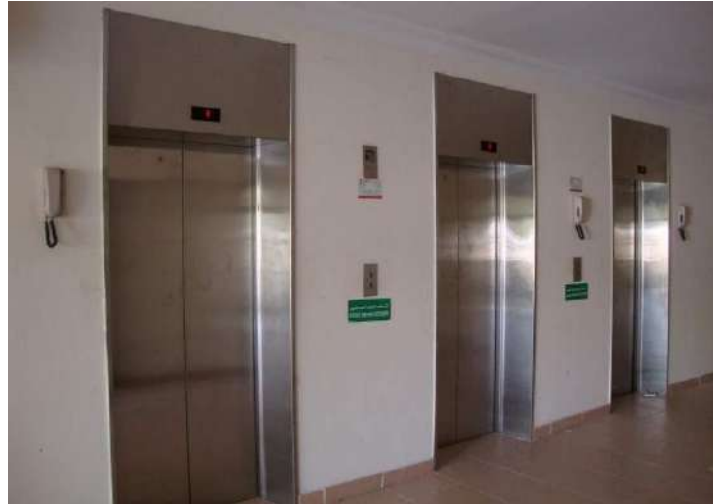
Units in Doha commercial building
