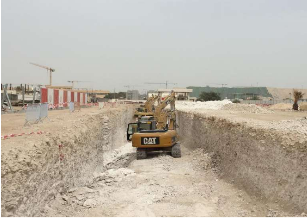
Excavation works at Duhail
