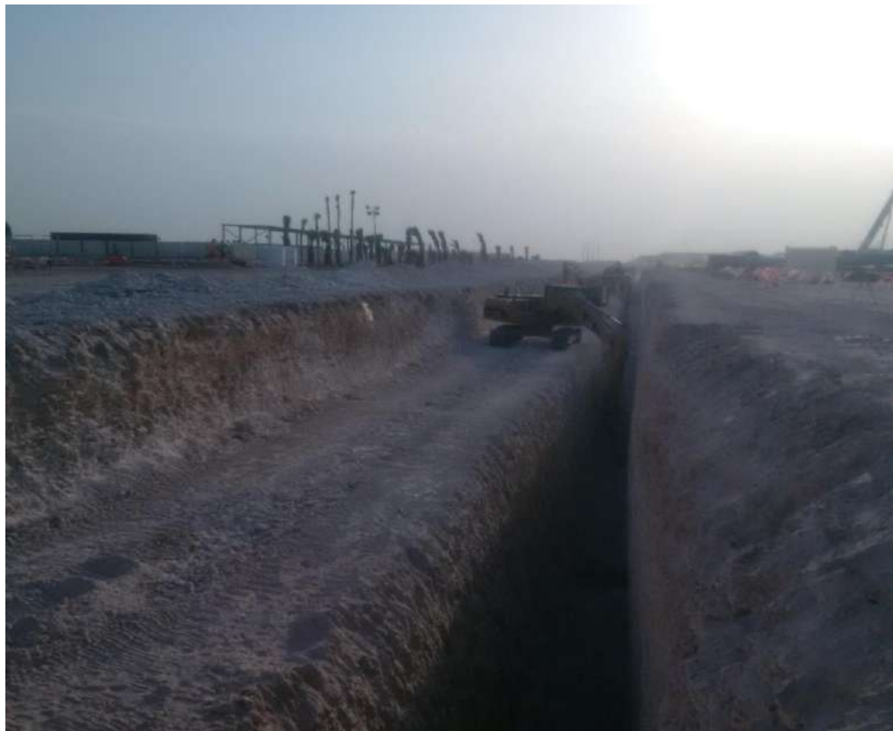
Excavation works at Duhail
