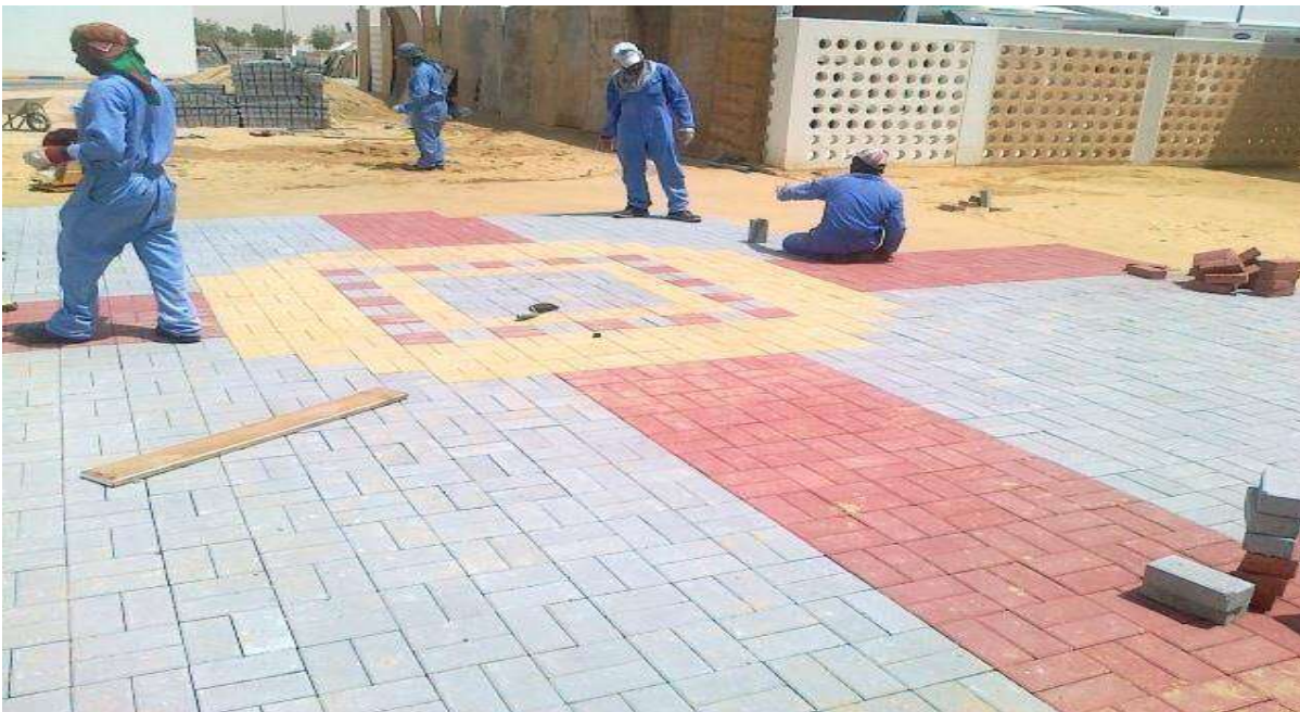
Beautification work at Al Khore Hospital
