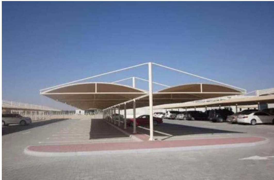
Parking Shed Rumailah Hospital – HMC
