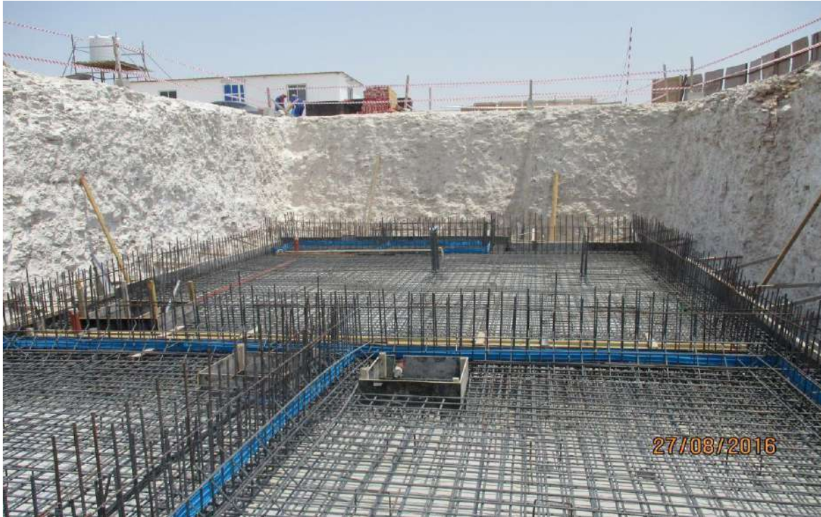
Hawqa Sportswear Manufacturing Factory – Foundation works
