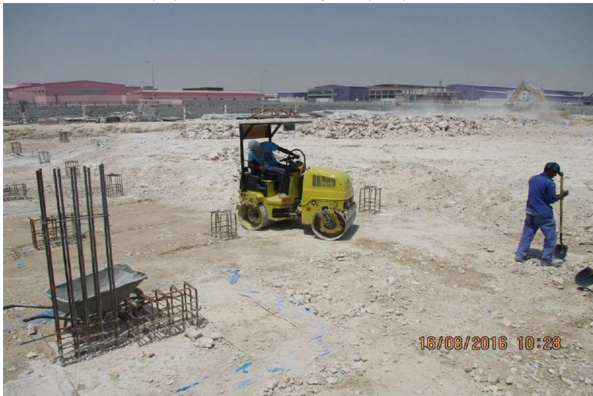
Hawqa Sportswear Manufacturing Factory – Foundation works
